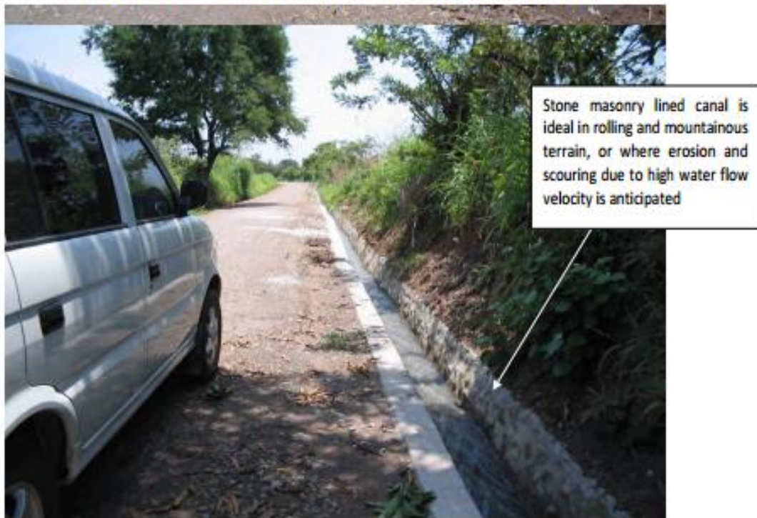
FMR with concrete/stone masonry lined canal. (ARCDP2)
