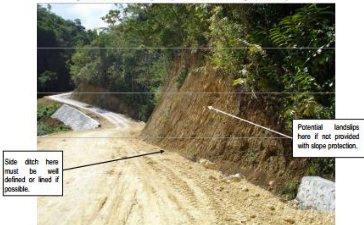
Damage on the road carriage way due to poor drainage.(ARCDP2)
