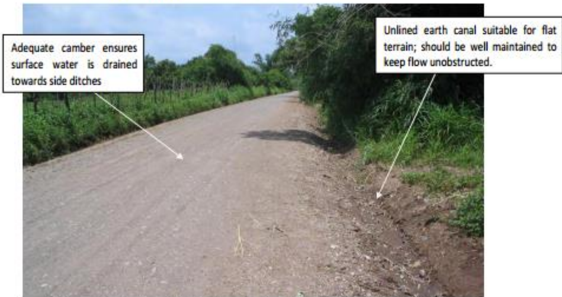
Well-constructed, well drained road with unlined earth canal. (ARCDP2)
